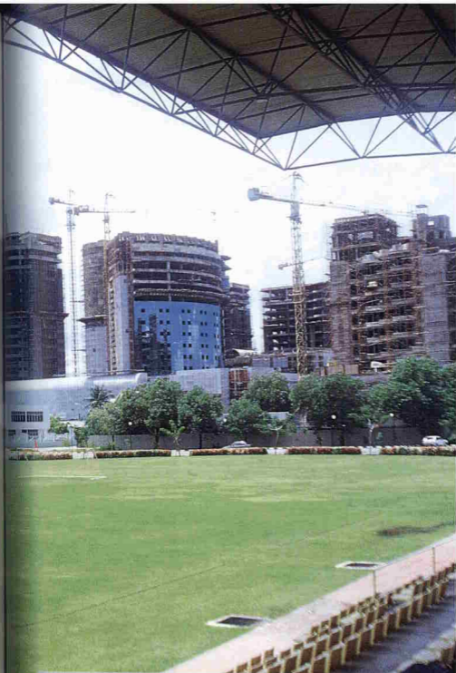
Front view of the new International Financial Centre, under construction in Labuan (IFOC)
